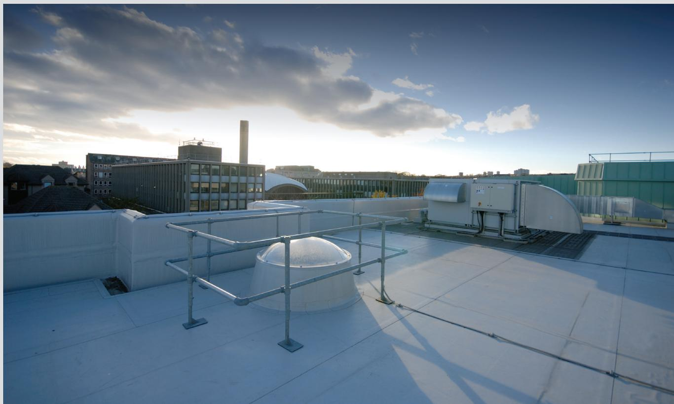
"The curator was concerned about the possibility of fire or water leaks," Richard recalls. "But Sarnafil had just introduced its Sarnacol 2162 polyurethane insulation adhesive, which meant there was no need for bitumen and hot works - perfect for this project. He was anxious for the project to go smoothly and thankfully it did." The Queen Mother Library's roof was also successfully refurbished, safeguarding its one million books and manuscripts.
