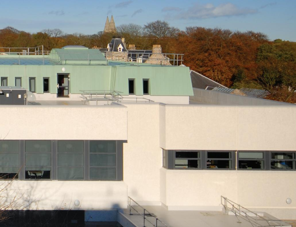
The roof of 'The Hub', Aberdeen University's dining, leisure and social facility is finished in Sarnafil copper patina, with Sarnafil Decor profiles which simulate the appearance of a traditional standing seam roof.
